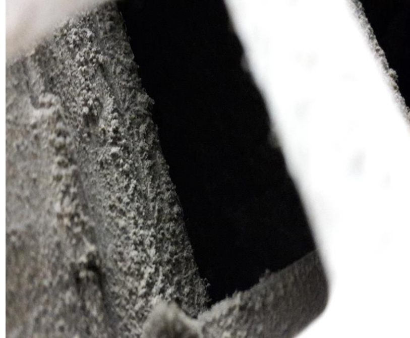
Ventilation flap filled with dust
